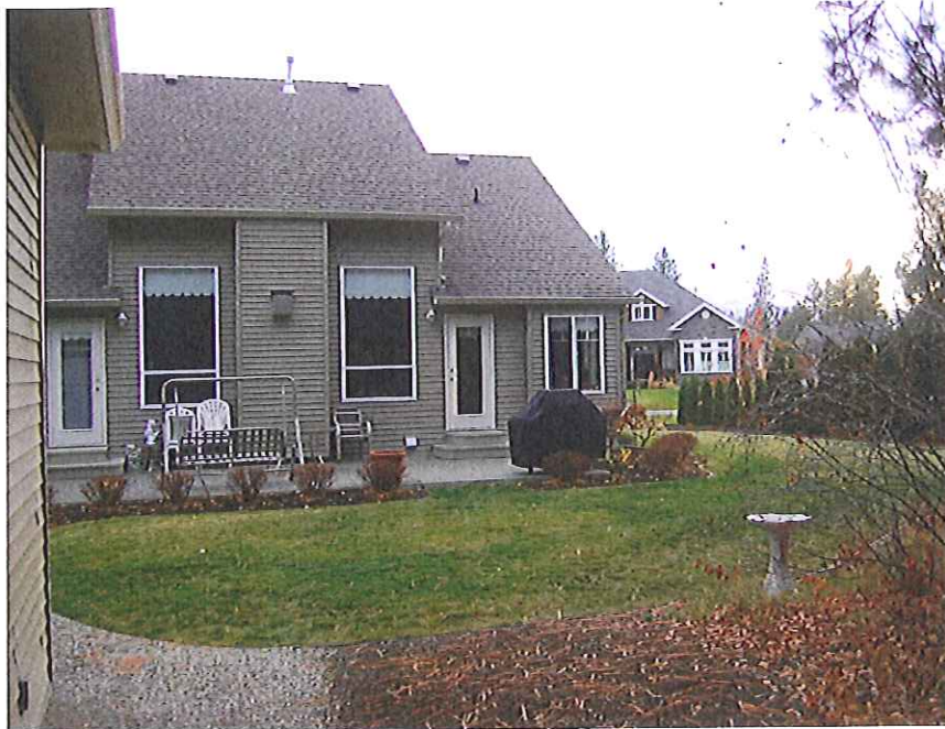
Rear of Main House (North facing)
