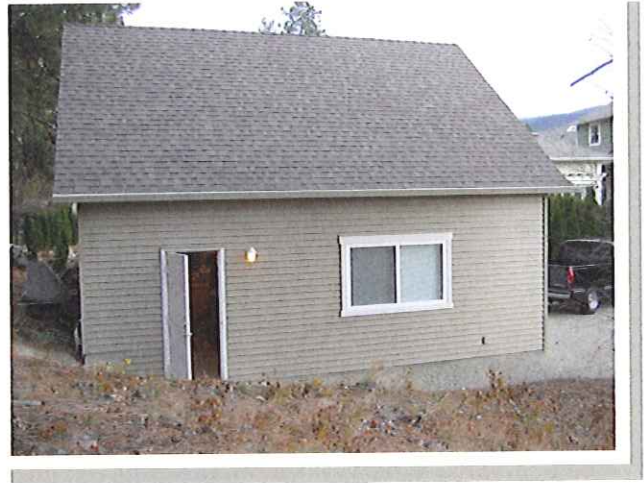
Auxiliary Building: Before Extension
