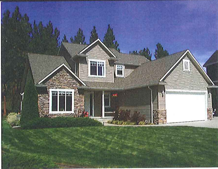
Front of Main House (South facing)
