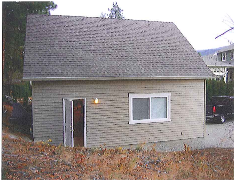
Side of Auxiliary Building (West facing)
